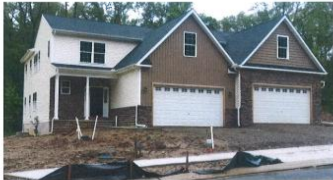
Twin homes under construction
