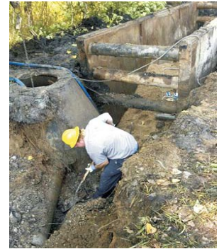
Sewer rehabilitation work underway
